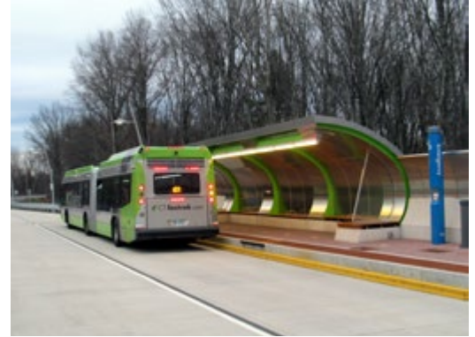
P-R4. Photo of a CTfastrak station
