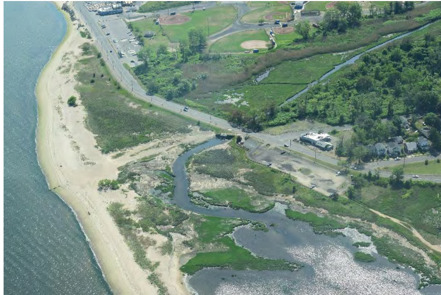
Photo 2-16: Old Field Creek
