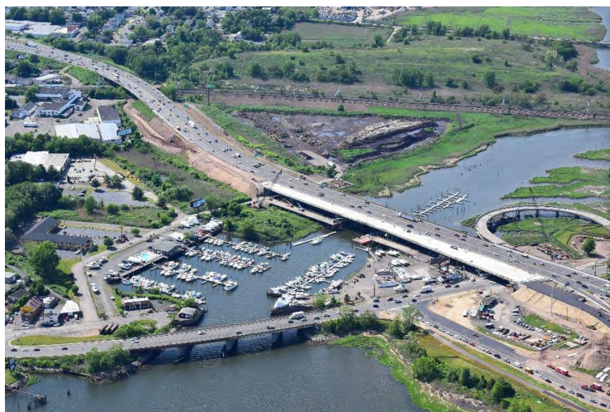
Photo 2-11: West River Crossing area including the I-95 and Kimberly Avenue bridges, the City Point Yacht Club facilities between the bridges, and the West Haven compost site upstream of the I-95 Bridge
