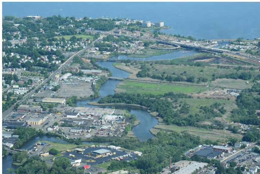
Photo 2-10: West River between New Haven (to left) and West Haven
