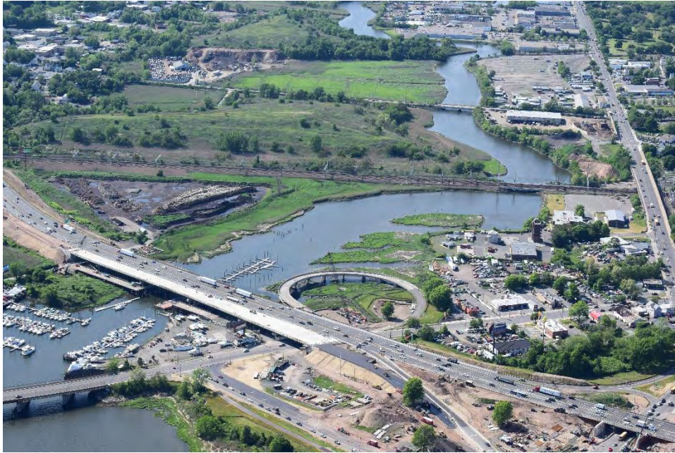
Photo 7-1: West River Looking Upstream; Compost Site to Left.
