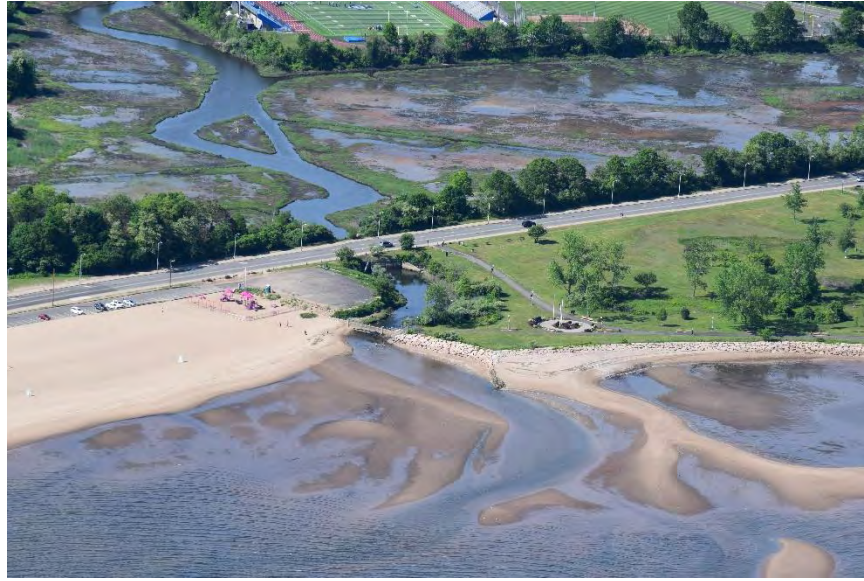
Photo 4-2: Cove River estuary; existing tidegates at Captain Thomas Blvd.; former pedestrian bridge and previous tidegate location at mouth of Cove River.
